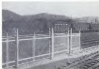
When unusual problems arise, Cyclone engineers can usually find a solution. This special Roller gate shown above covers a span of approximately 70 feet.
